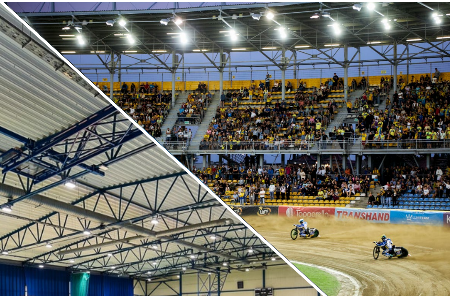
Sports hall lighting at the Sports and Recreation Center of Grodzisk Mazowiecki, Poland
