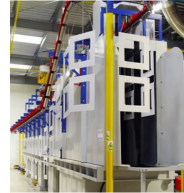
Ecological powder paint shop
